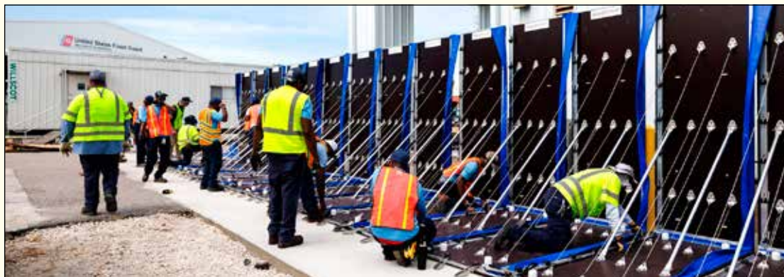
One of the completed SPAR projects, an AquaFence installed to protects a vital wastewater lift station near Albert Whitted.
